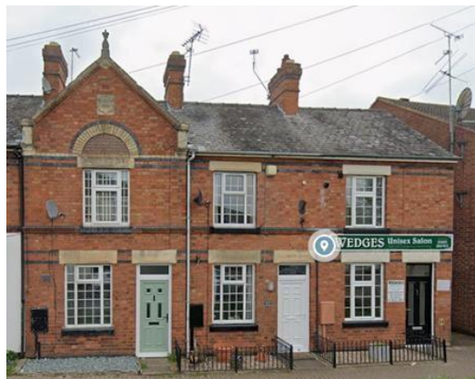
56-60 Main Street. A red brick terrace with contrasting buff and dark brick ornamentation, including a tiled semi-circular segment in the eaves gable below a datestone that reads '1889'
