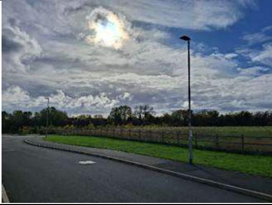
Image 4. Within Site (facing north – eastern boundary on RHS)
