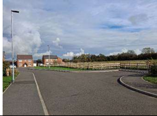
Image 5. Facing West (within site at northeast boundary)
