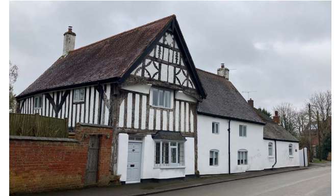
Figure 15: White timber framed structure buildings
