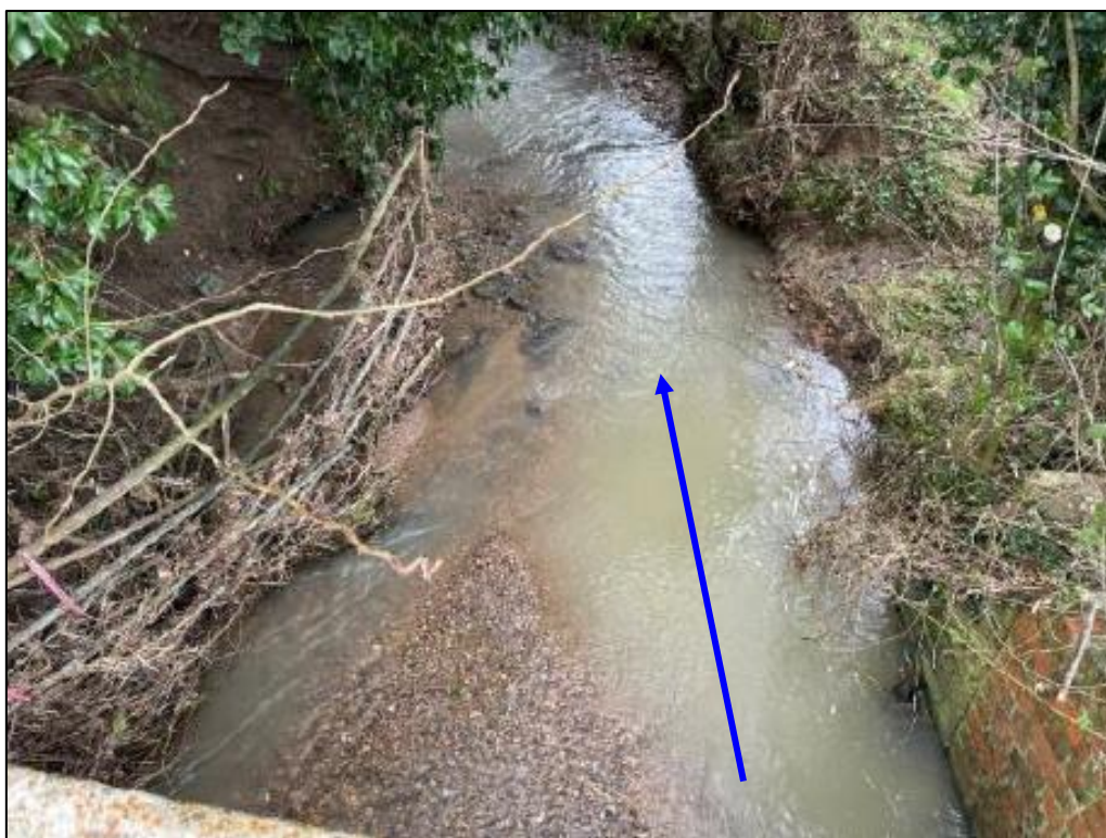
Photograph 7-7: Silt deposition within the Glooston Arm on outlet of the Harbrough Road Bridge culvert looking downstream following the flood event 3
