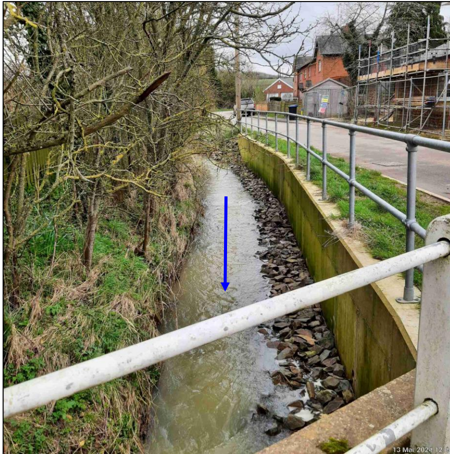
Photograph 7-6: Bank reinforcement upstream of Harbrough Road Bridge looking eastwards towards Cranoe Road
