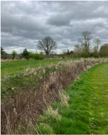
Figure 82: A swale incorporated as part of the SuDS strategy and 'green buffer' at Hursley Park.
