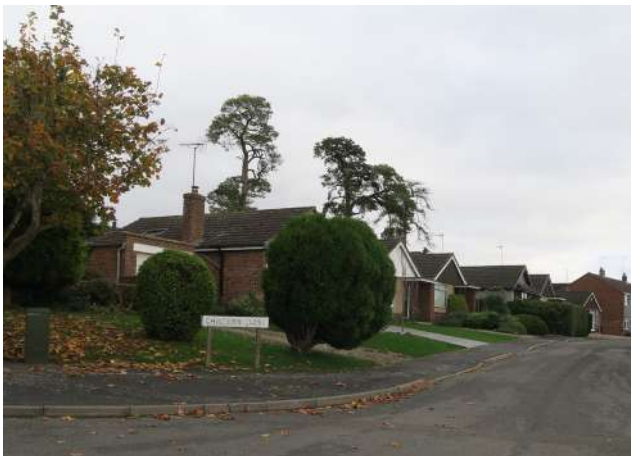
Figure 64: Bungalows on Chiltern Close
