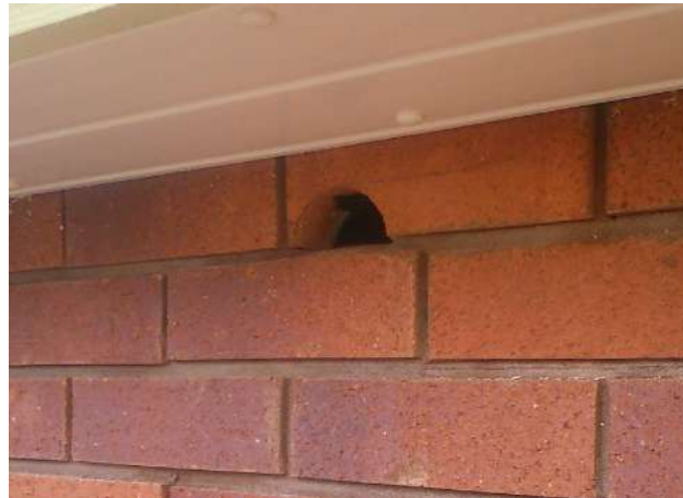
Figure 26: Example of a Swift brick under an eave
