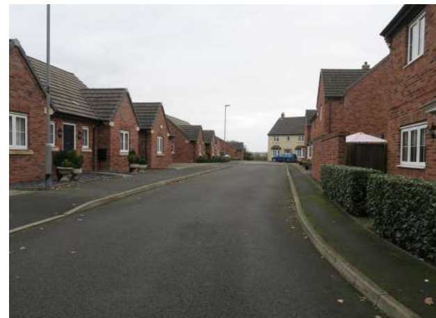
Figure 72: Bungalows and two-storey house, Centenary Close
