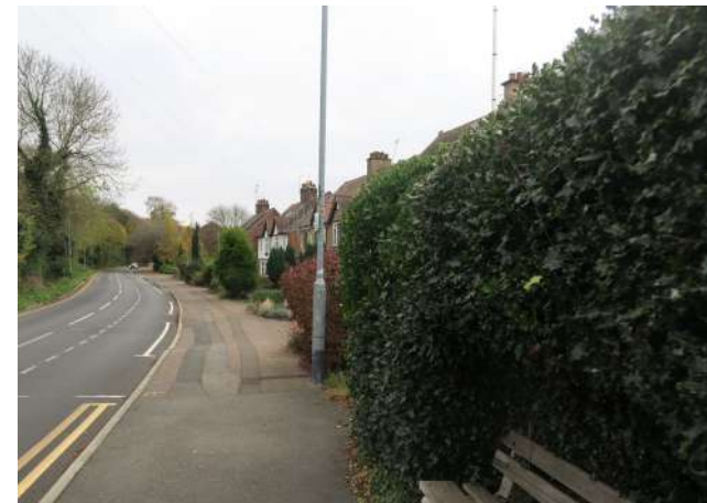
Figure 52: Front gardens screened by landscaped boundary hedges, Great Bowden Road
